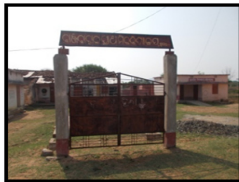
Figure-11: Partially constructed boundary wall in Banji bahal Primary School.
